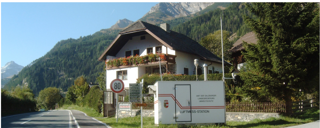
Measuring station for immission monitoring
